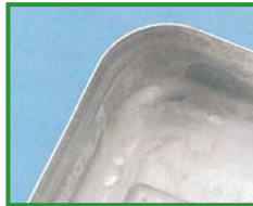
Material attack. Cause: Alkaline cleaner
