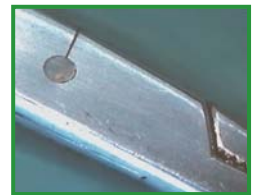
Fracture at hinge pin
